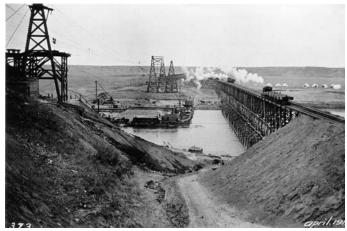
Water has always been important to the Bassano region. Without it, there would be few people and little commerce. In 1910, the CPR began construction of this dam 6 km southwest of Bassano to open up the region. In 1935, a group of farmers bought the Bassano Dam and canal system from the CPR, forming the Eastern Irrigation District (EID) that provides water in an area larger than the province of Prince Edward Island. Virtually all
